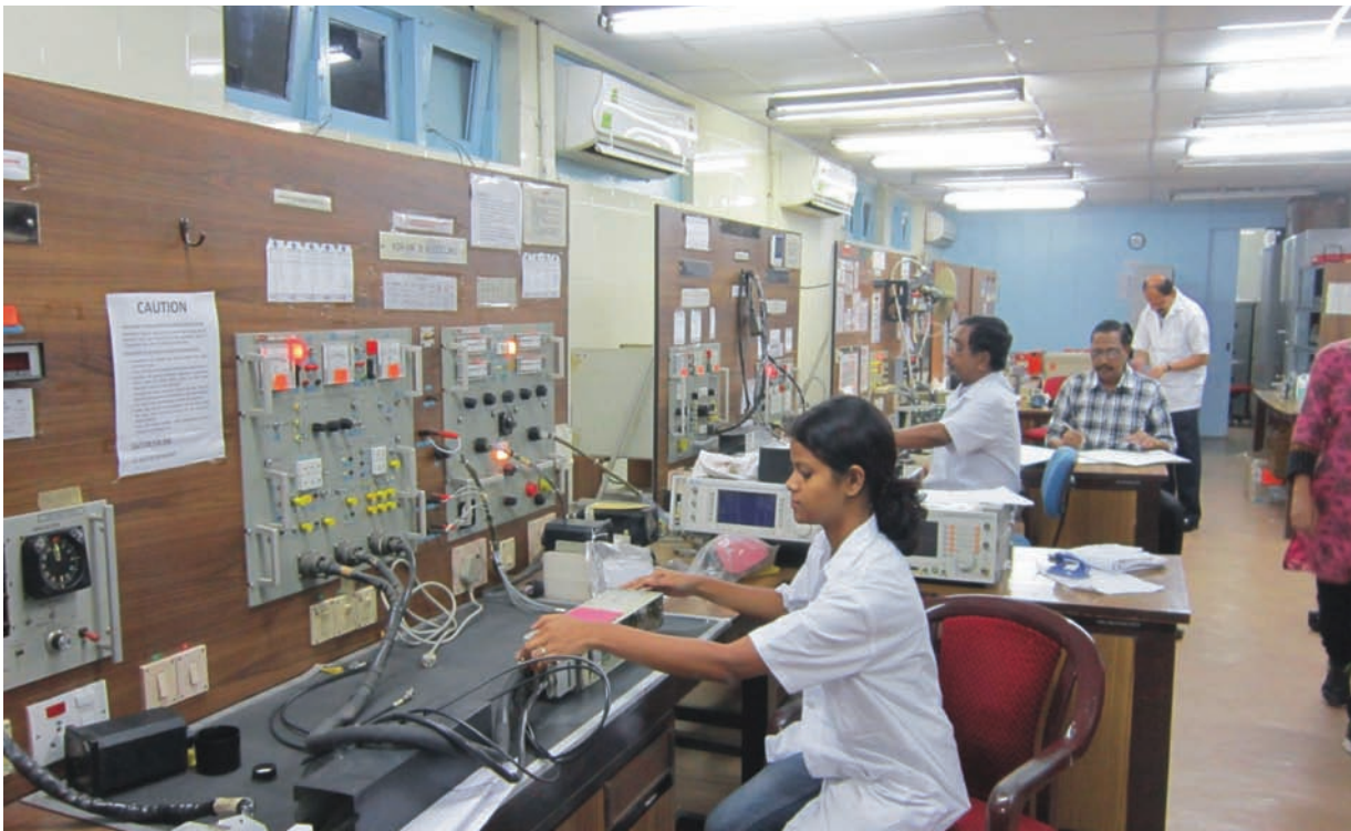
Battery Maintenance in approved Battery charging room
