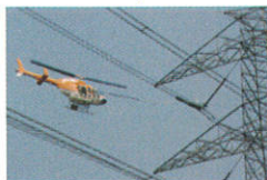
2008 Power Line Maintenance for PGCIL
