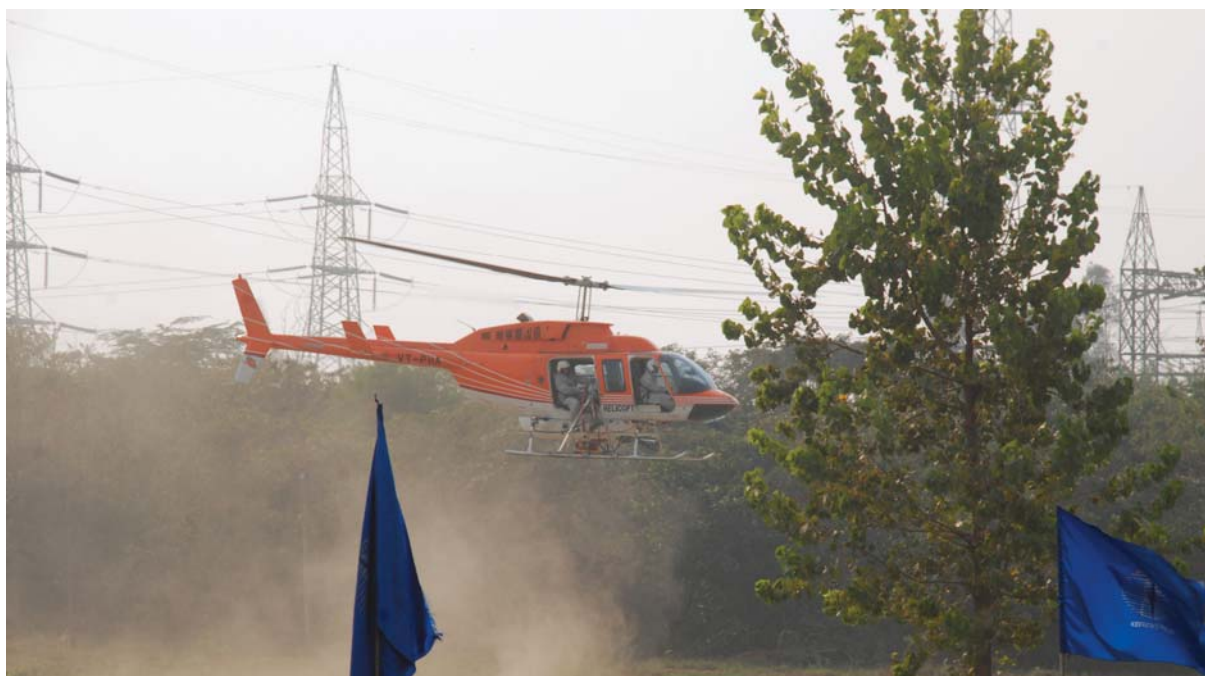
Hotline Washing of Power Insulators
